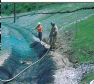
Slope interceptor ditch on steep slopes
